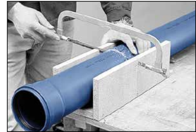
Cutting to length with a fine-toothed saw (FIGURE 17)
